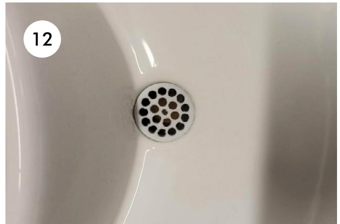
12. To prevent particles from getting into the urine hose and clogging the drain, please insert the enclosed strainer into the liquid outlet of the seat part. The strainer surface must be facing upwards.
